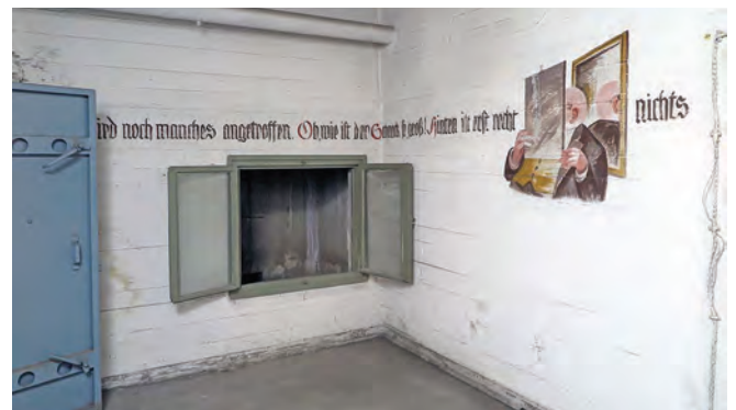
General view of air-raid shelters, with hatch to emergency exit ladder in the back wall. Photo Clive Penfold
